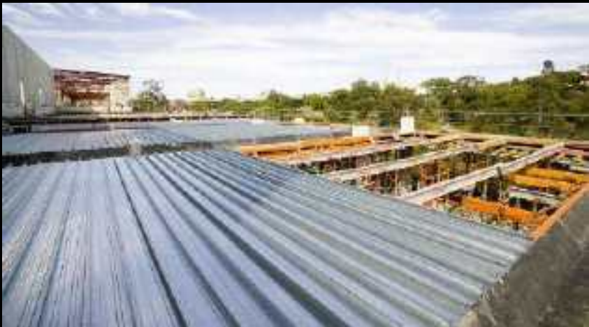
Reinforced concrete slab with metal formwork
